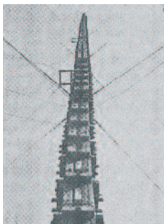
The first lightning collector tower on Mount San Salvatore, a 70 m timber mast that used to be the Berne TV transmitter.
