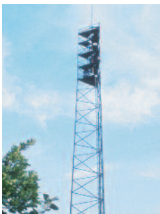
In 1950 the second 70 m lightning collector tower was erected on mount Pian San Carlo nearby.
